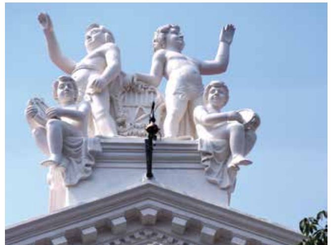
The marble cherubs on the rooftop after the restoration
